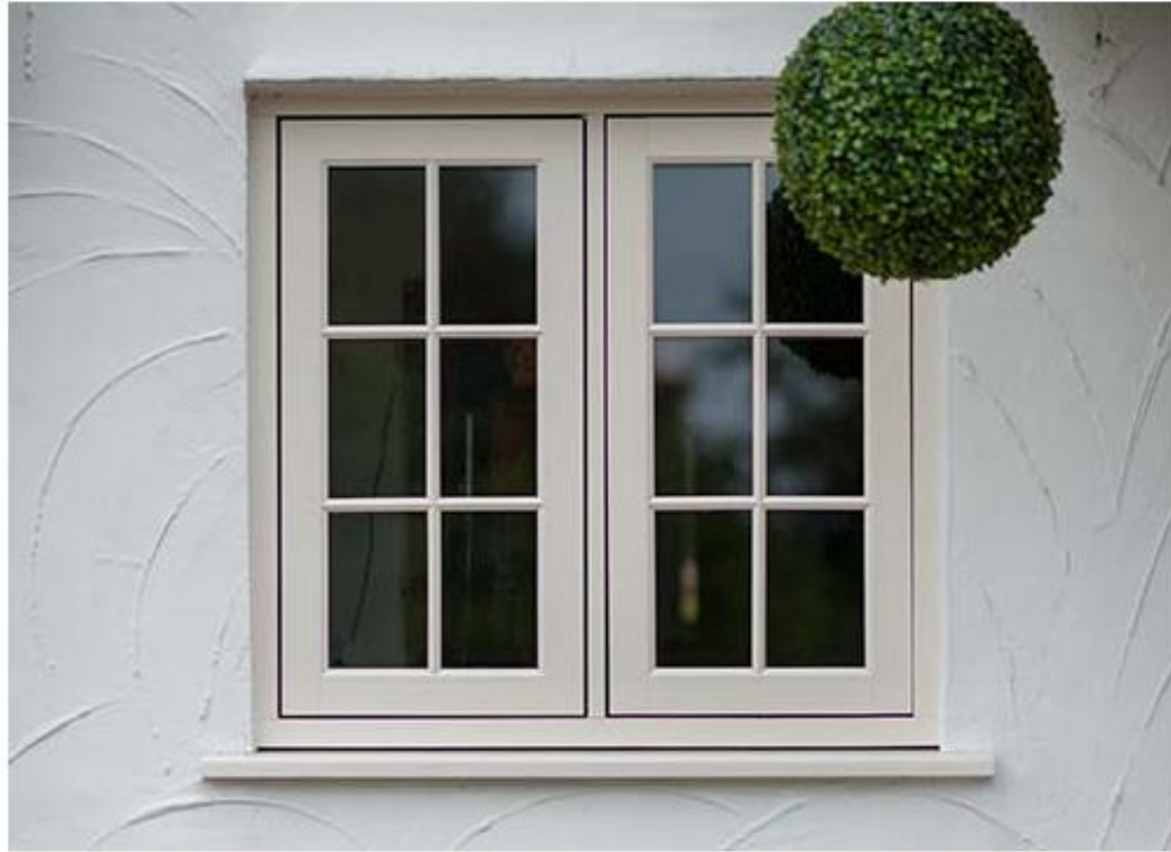
Illustrative example of proposed UPVC Flush casement windows with Georgian Bars to be provided in white at 15a Cliff Avenue.
